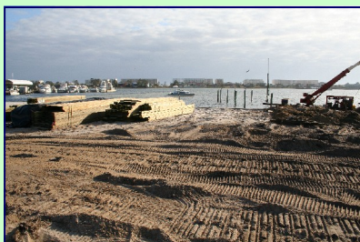
Installation of the Seawall
