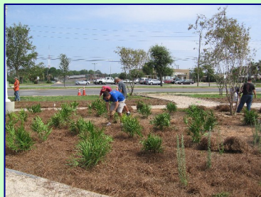
Landscaping in Progress
