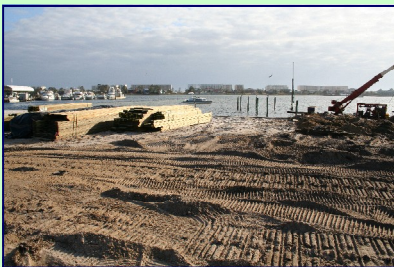
Installation of the Seawall
